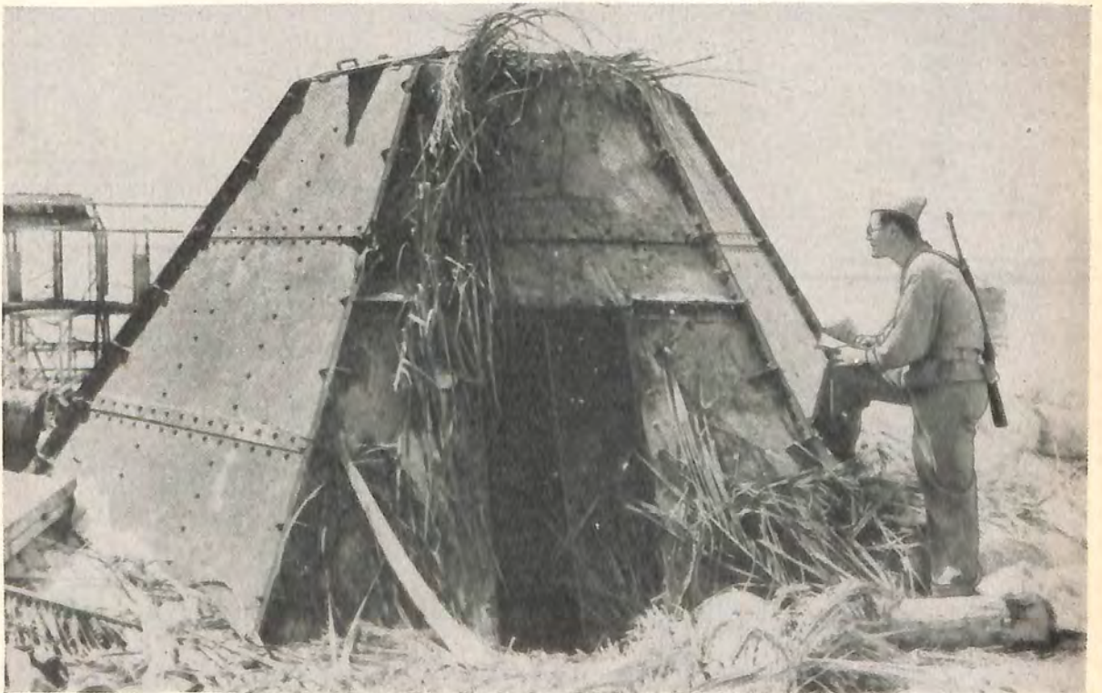
Figure 145. A hexagonal steel pillbox.
